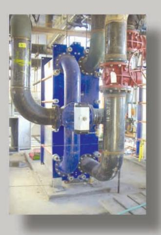
The Automatic Back-flushing System 4way valve uses reversed water flow to clean the plates while the heat exchanger remains on-line.
