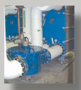
This HX-type valve fits easily into plate and frame heat exchanger piping and eliminates the need for manual cleaning.
