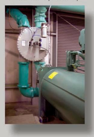
The ATB System 4-way valve reverses the condenser water flow for about 30 seconds every 6 hours.
