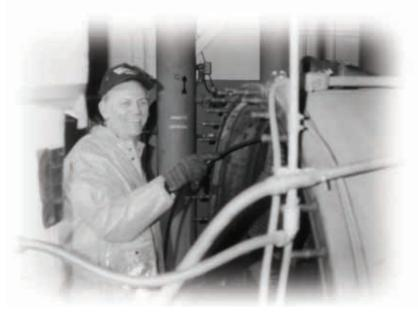
This outdated method of cleaning tubes cannot fight the scale and slime that start forming immediately after equipment start-up.
