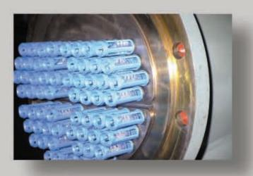
ATB System brushes and baskets, the key to a strong system payback, installed in a condenser tube sheet.
